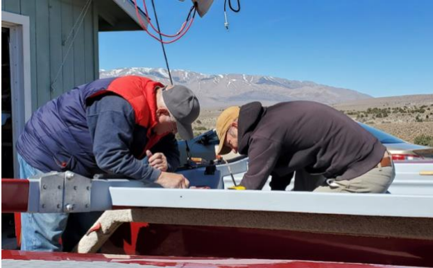
New cockpit drains—Guy’s help has been instrumental
