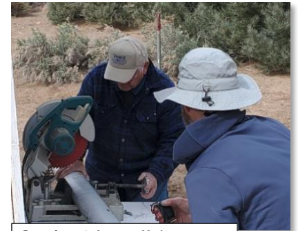
Cutting 2 feet off the mast
